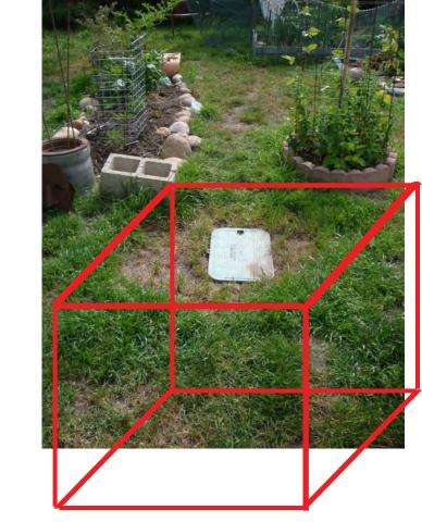
Downspouts and drains from the roof and patio lead to a 6' deep, 4'x4' gravel-filled pit in the backyard. A sump pump is inserted into a pipe (covered by the valve box) and the water is used to irrigate the garden when it fills up and in drier months.
